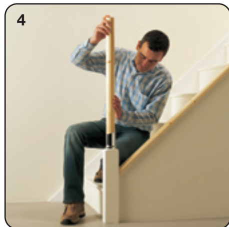
4 After measuring your post to the correct length, fit and secure the posts in place. Repeat for all newel posts.
