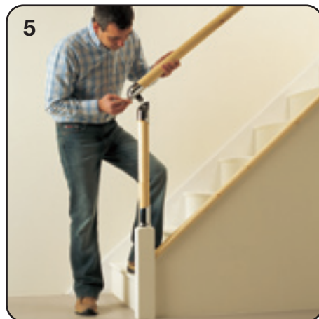
5 Attach the handrail using the bottom connector.
