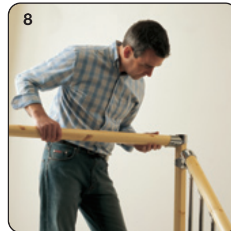
8 Begin fitting appropriate landing balustrading.
